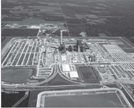
Aerial View, Late August 2010
