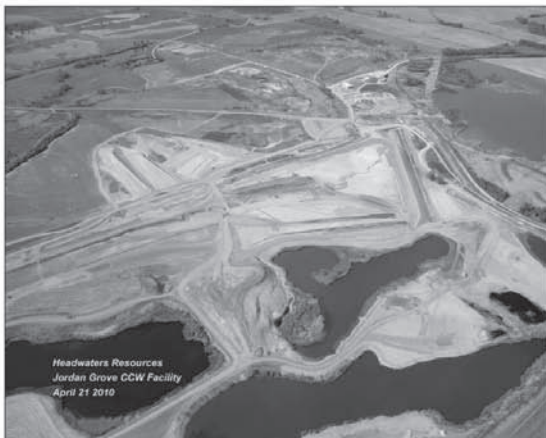
Jordan Grove CCW Disposal Site, April 2010
